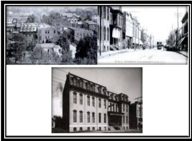
FIGURE 1: ST. JAMES HOTEL AT 228 NORTH MAIN STREET
